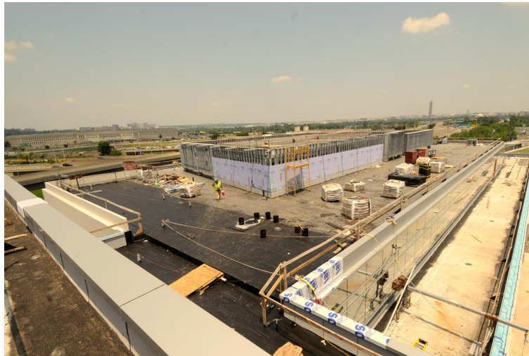
Figure 4 – View of Penthouse from Roof (Courtesy of Davis)
