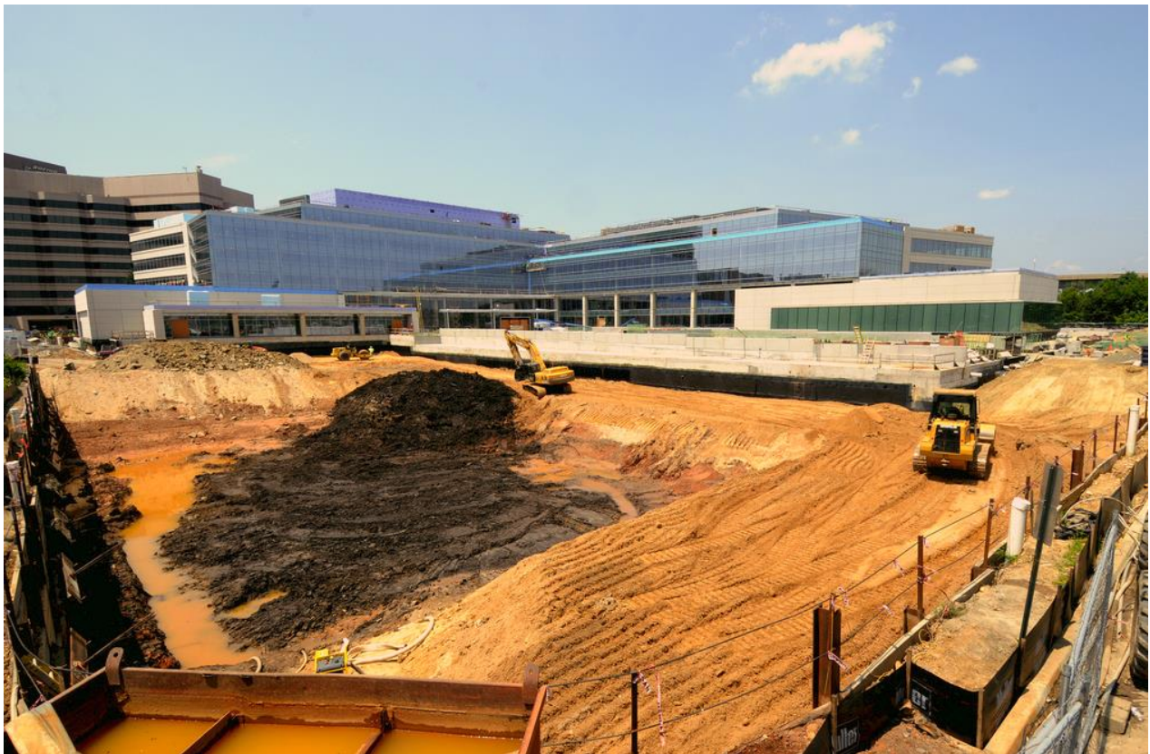
Figure 2 – Excavation for Future Addition (Courtesy of Davis)
